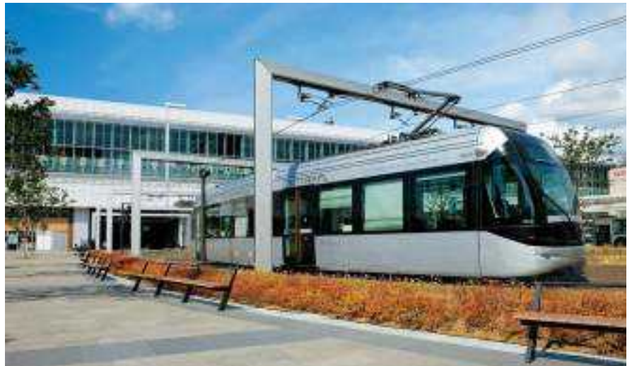
路面電車南北接続事業で誕生した富山駅前の軌道空間とLRT Space created in front of Toyama Station by connecting the North and South streetcar lines and LRT
